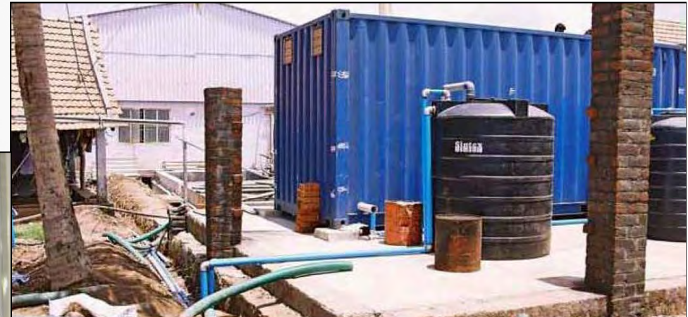
DYE WATER TREATMENT BUILDING CONSTRUCTED AROUND THE CONTAINER
