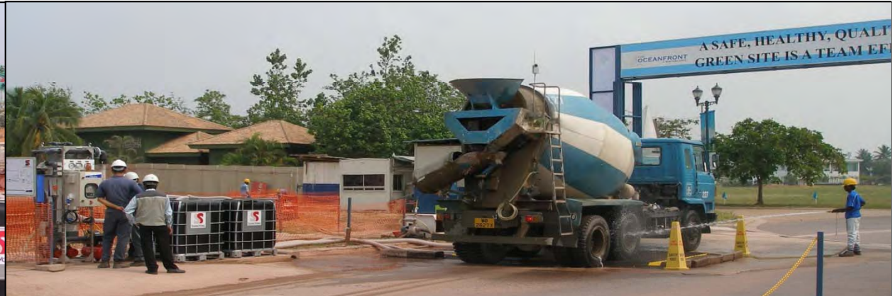
Recycling of silty water with MU02-8 System at 8 m 3 /hr
