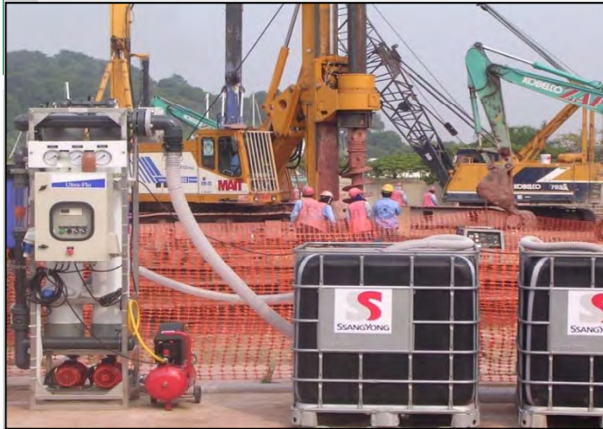
Recycling of silty water with MU02-8 System at 8 m 3 /hr
