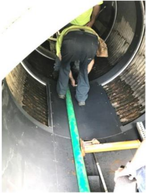
(Sadsbury, USA) CMP Invert Repair
