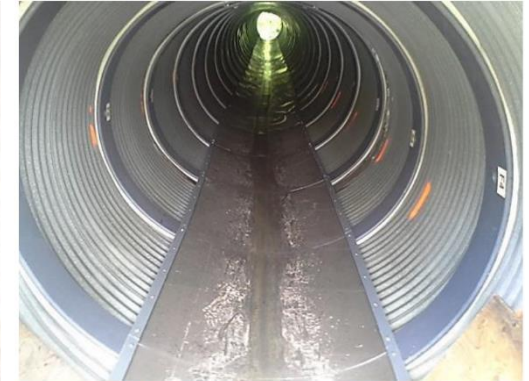
Rib and Trough Installed
