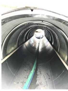
Rib and Trough Installed
