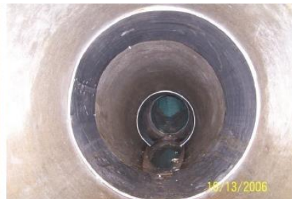
Grouting Sleeve ™ instalada
