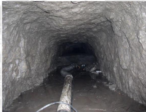
(Kingston, USA) Horseshoe tunnel rehabilitation
