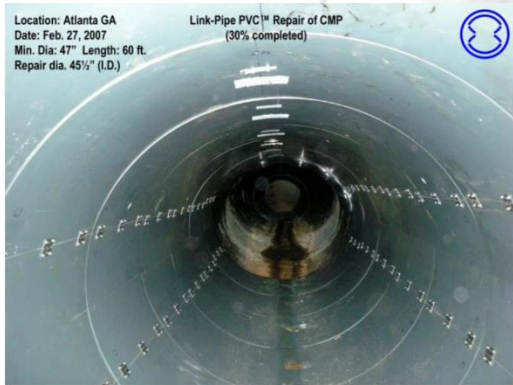
(Atlanta, GA) Continuous Installation Link-Pipe PVC
