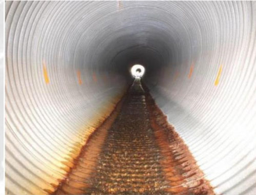
(Ontario, CA) Invert repair of corrugated metal pipe.
