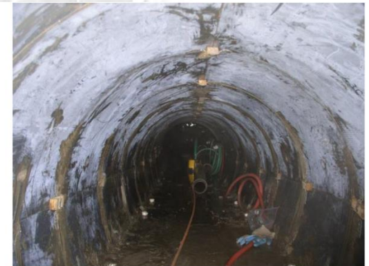
Link-Pipe Horseshoe Shape PVC™ Installed
