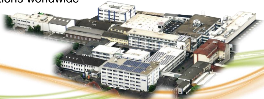
Headquarter, administration, and production sensors + automation
